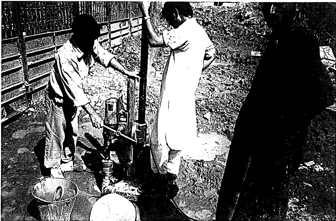
Photo. 5.6: Coring works in progress. In the background inhospitable environment is quite visible.
