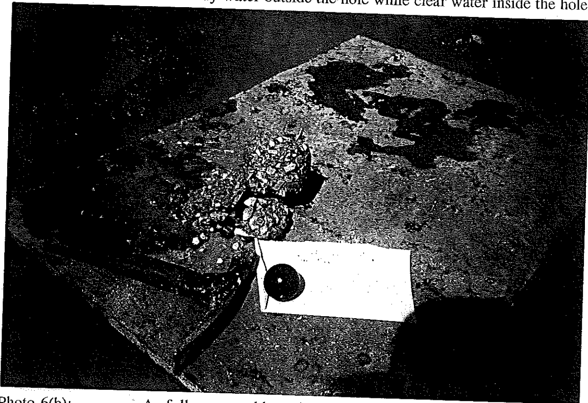
Photo.6(b): As full core could not be extracted and further coring resulted in disintegration of concrete, hence only slush material was removed.
