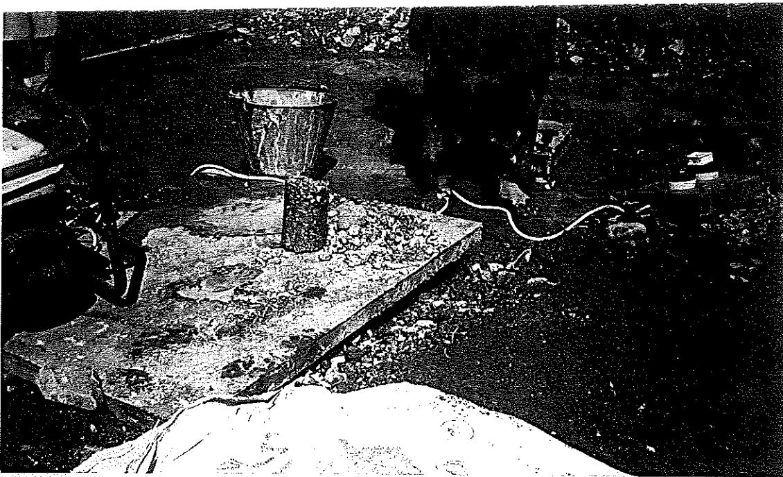
Photo.7 (a): Core 2 could only be drilled upto 150 mm below the clear cover level. Further coring works were abonded after disintegration of concrete Core .
