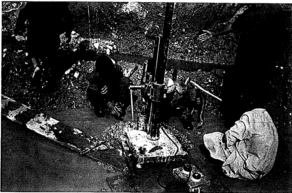
Photo.5.8: Coring works in progress. In the background in hospitable environment is quite visible.
