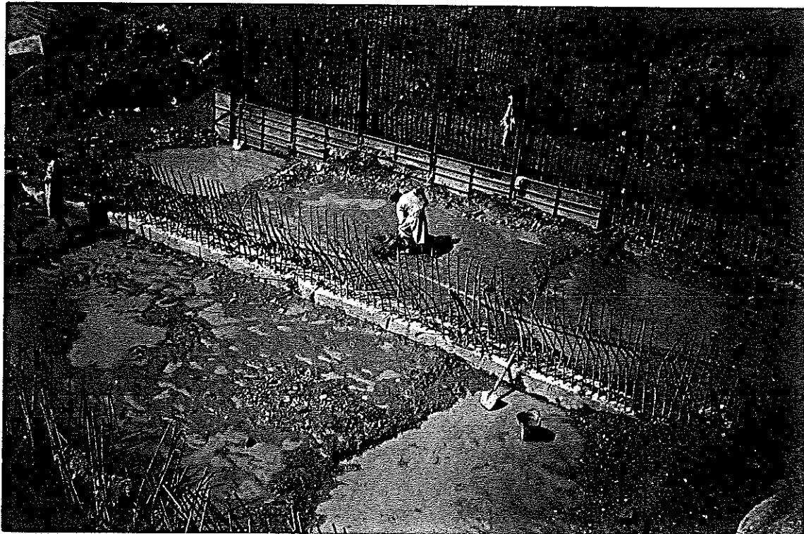
Photo. 5.2: Another view of the site on 01-10-1998 showing clearing works in progress.
