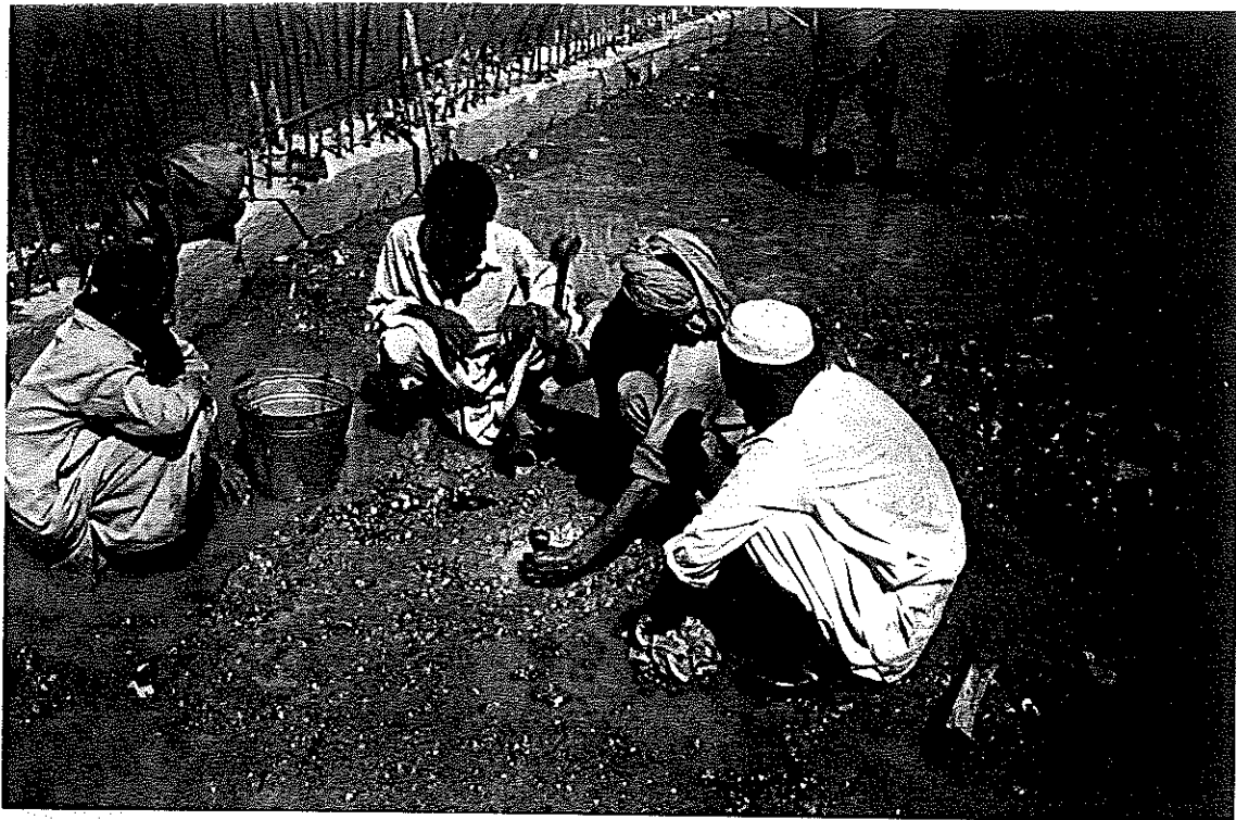
Photo. 5.3 Work in progress for exposing the reinforcement, and in the background debris being removed from the base slab.
