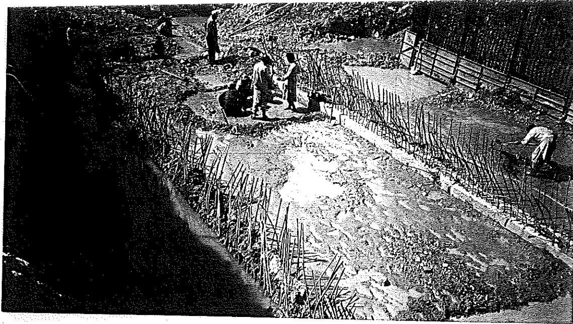
Photo.5.1: A General view of the site on 01-10-1998 at 11:00 am. The site was unsuitable for Coring works as can be seen. Upto two feet mud covered the base slab of the box culvert.
